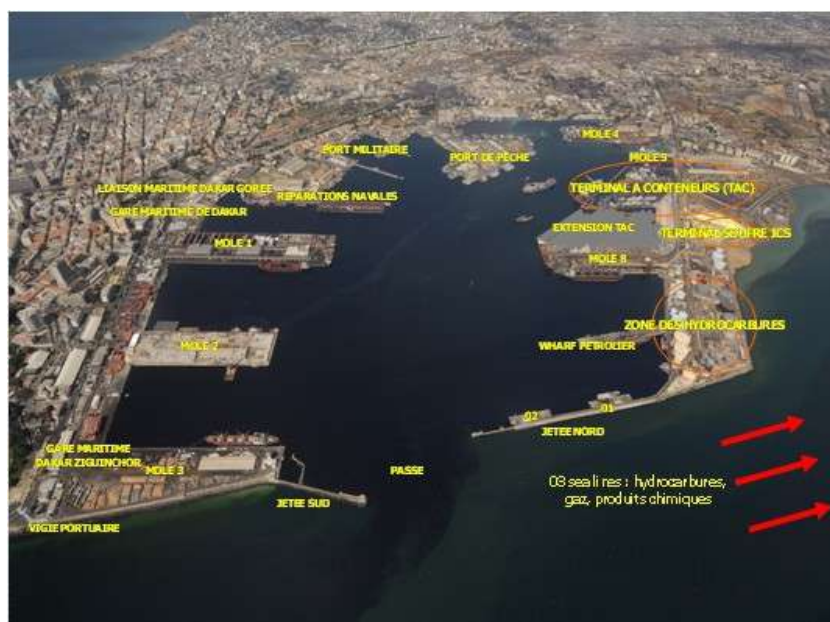
Figure 25.1: Port de Dakar.
